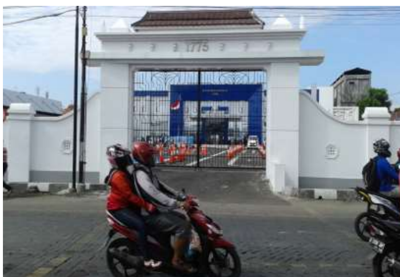
Figure 4.1 The New Building of the Administrative Organizing Unit SIM (SATPAS) Semarang City
